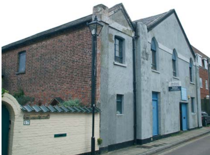
Figure 2: Frontage to Nile Street showing altered fenestration
