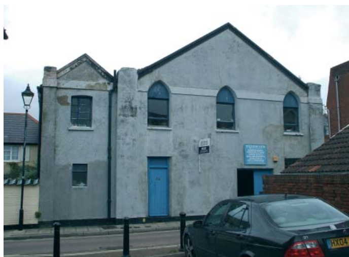
Figure 5: Front elevation of existing building
