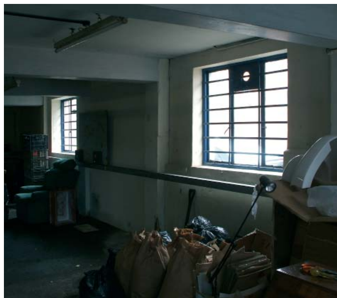
Figure 3: Inside showing concrete floors and beams and metal windows
