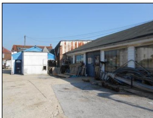
Figure 1: View of the site looking north
