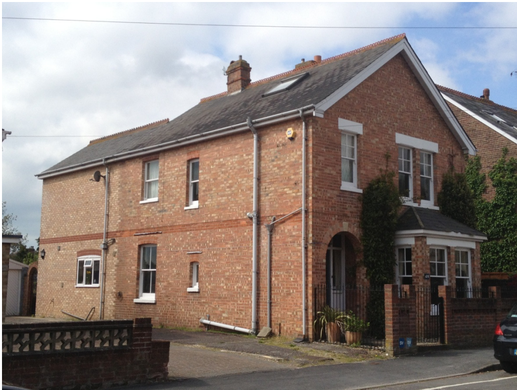
Fig No.1 – Image of Existing Building
