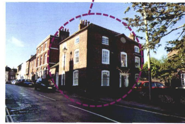
Three storey, red brick with hipped roof.
