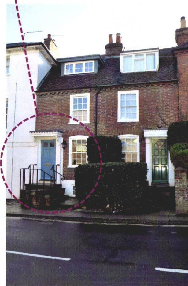
Stepped entrance with railings.
