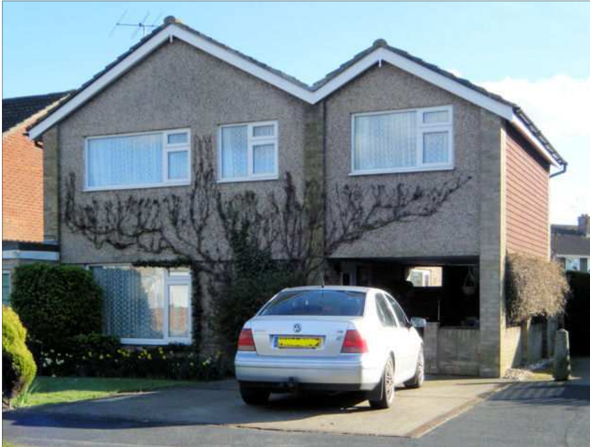
Front of No. 19 Luard Court with two storey side extension
