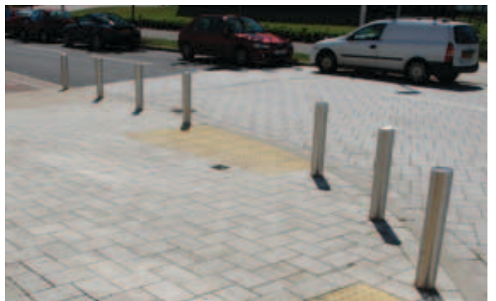
Tactile paving provided at defined pedestrian crossing points to guide the visually impaired
