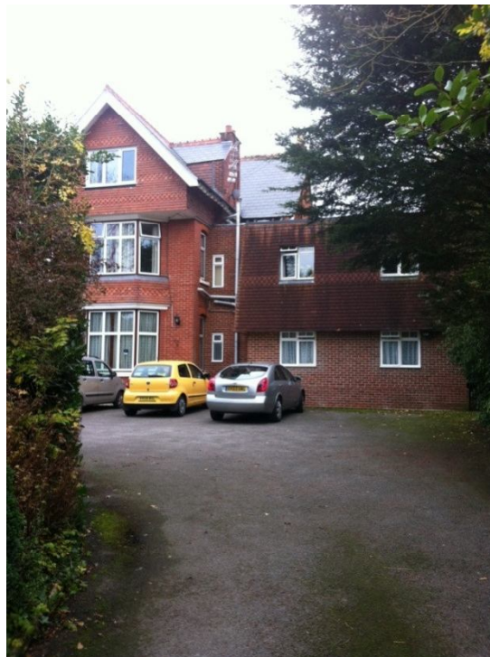
Image 7: View from New Brighton Road, showing existing East wing.
