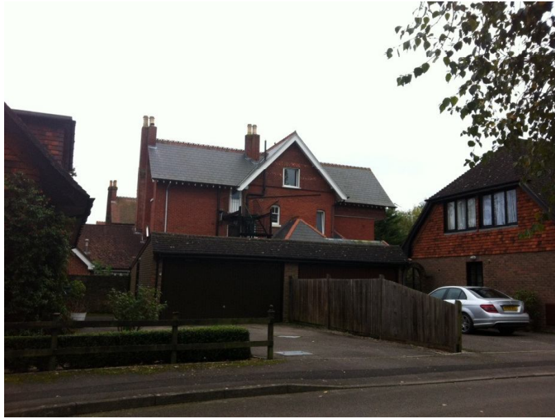
Image 6: View from Silvertrees, showing external fire escape.
