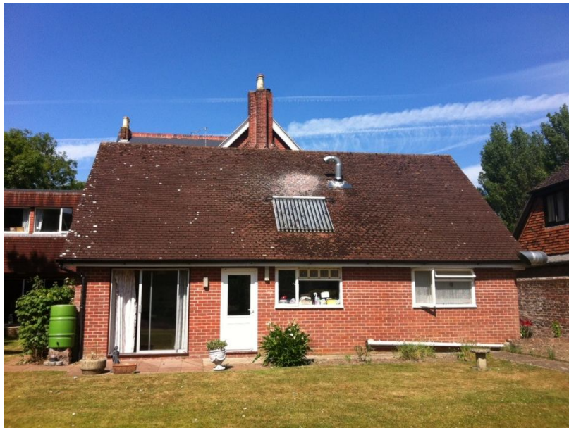
Image 5: Existing kitchen extension, to be demolished
