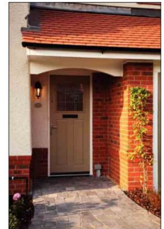
Photo 7: Tile roof porch
