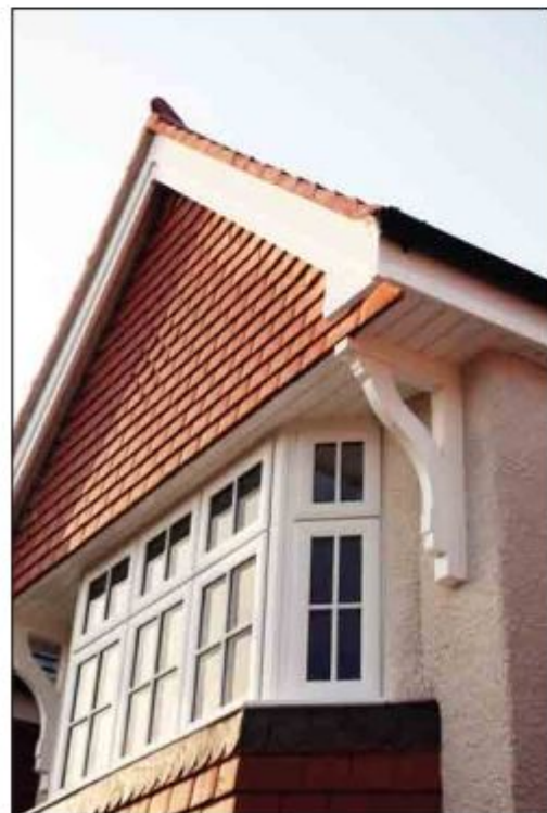
Photo 3: Tile hung gable end
