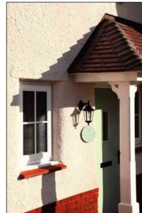
Photo 6: Timber post porch
