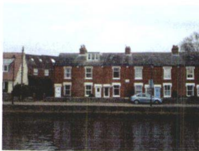
Existing West facing Dormer opposite Emsworth Basin.
