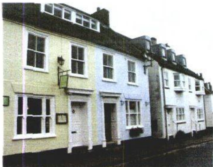
South Street, Emsworth. Light coloured finishes are characteristic of this row of houses in the historic core.
