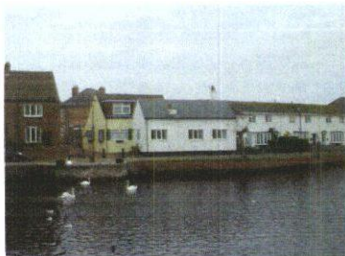
Existing West Facing Dormer opposite Emsworth Basin.
