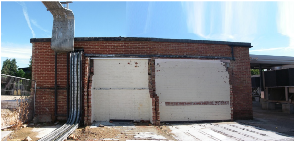
Fig. 2 - Existing Substation Building
