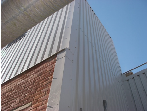
Fig. 1 - Surrounding Buildings on Pfizer Site
