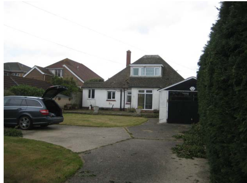
Street facing elevation to existing house at No 76 Southwood Road
