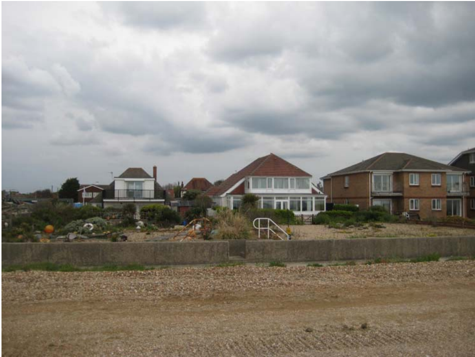
Photographic view of the rear of 76 – 80 Southwood Rd looking North as existing
