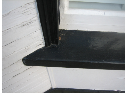
Fig 4– Existing ground floor window cill and side reveal to window frame.
