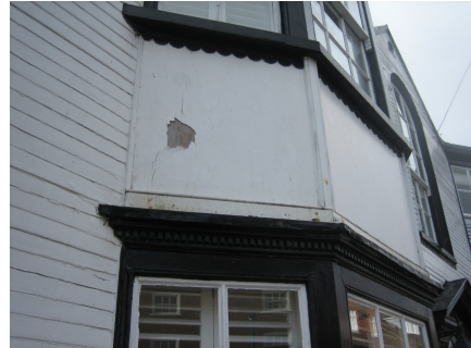
Fig 5 – View of existing upper plywood face to bay along with window head and first floor cill.
