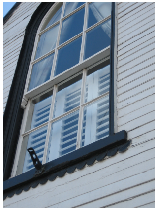
Fig 6 – Existing central window showing leadwork under cill and existing projecting frame abutting the cladding.
