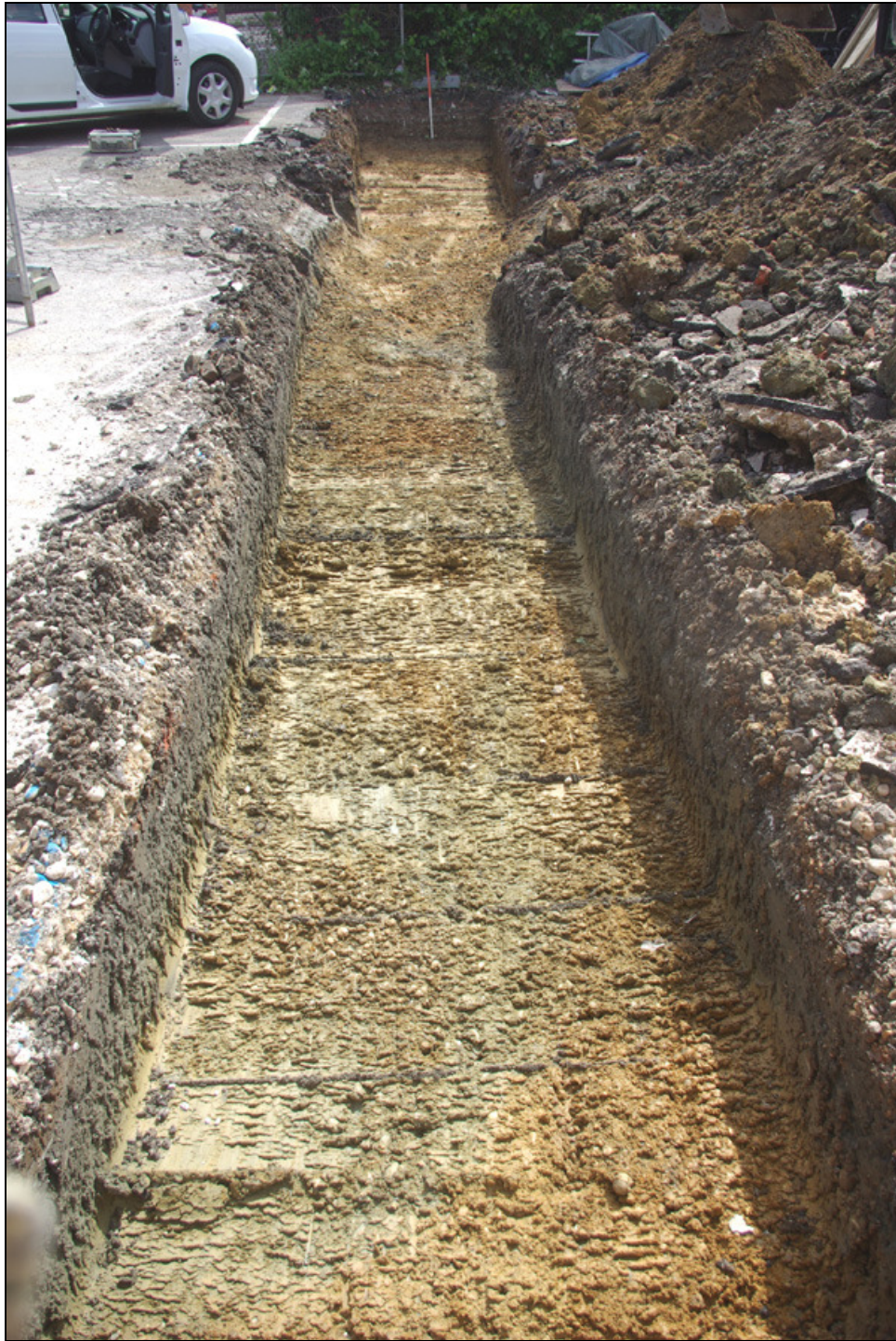
Figure 3 The investigation trench looking east. The scale is 1m.
