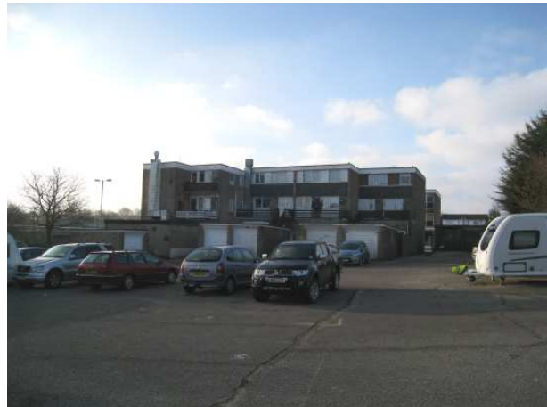
Units 1-4, viewed from the rear parking area (northeast)
