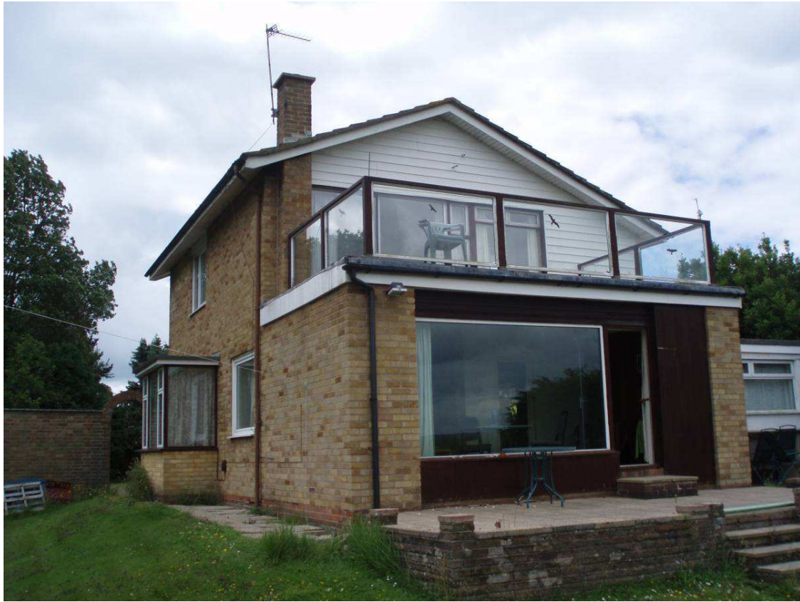
Photo 5 – View looking towards the northern gable and balcony also showing east elevation & bay.
