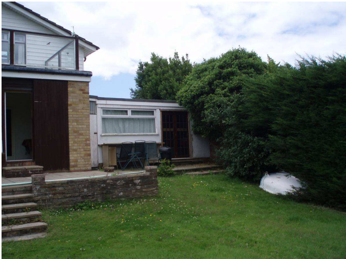
Photo 6 – View looking south-west with the western boundary to No. 6 on the right.
