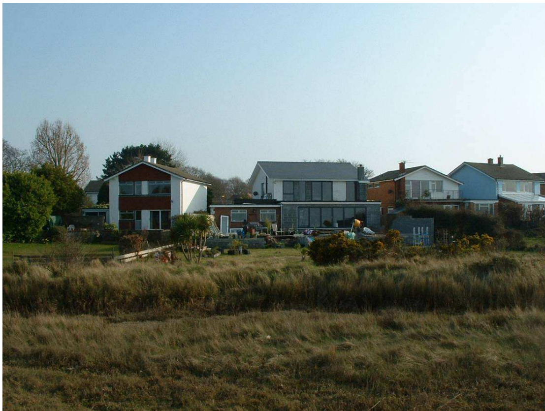
Photo 10 – View from foreshore with Nos. 6, 7, 8 & 9 from left to right.
