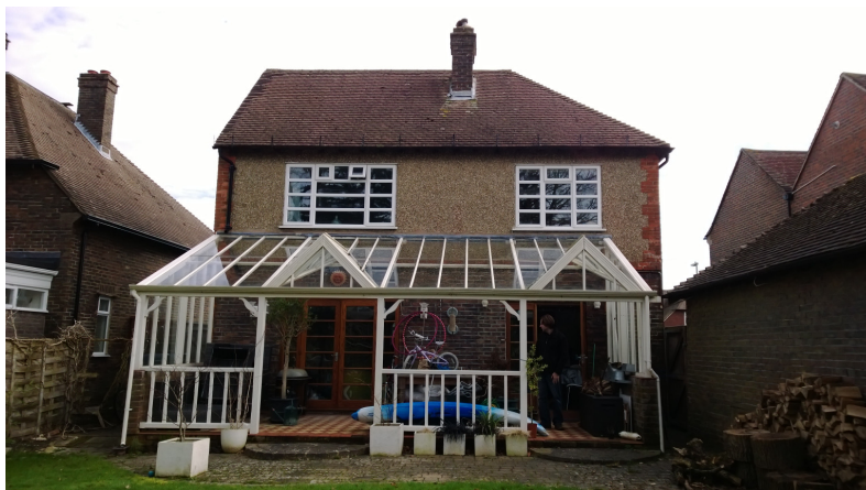
Rear veranda of our site.
