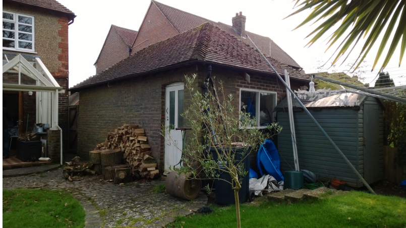
Garage to our site property.
