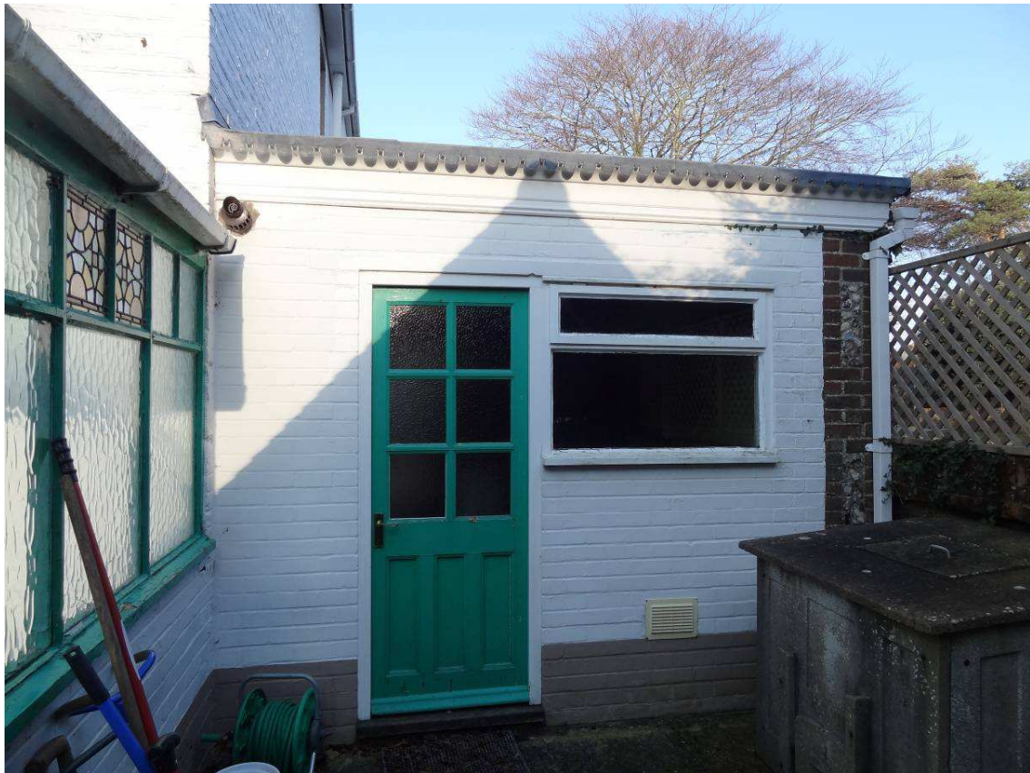
Photo 7 – Rear of existing side extension to be demolished.
