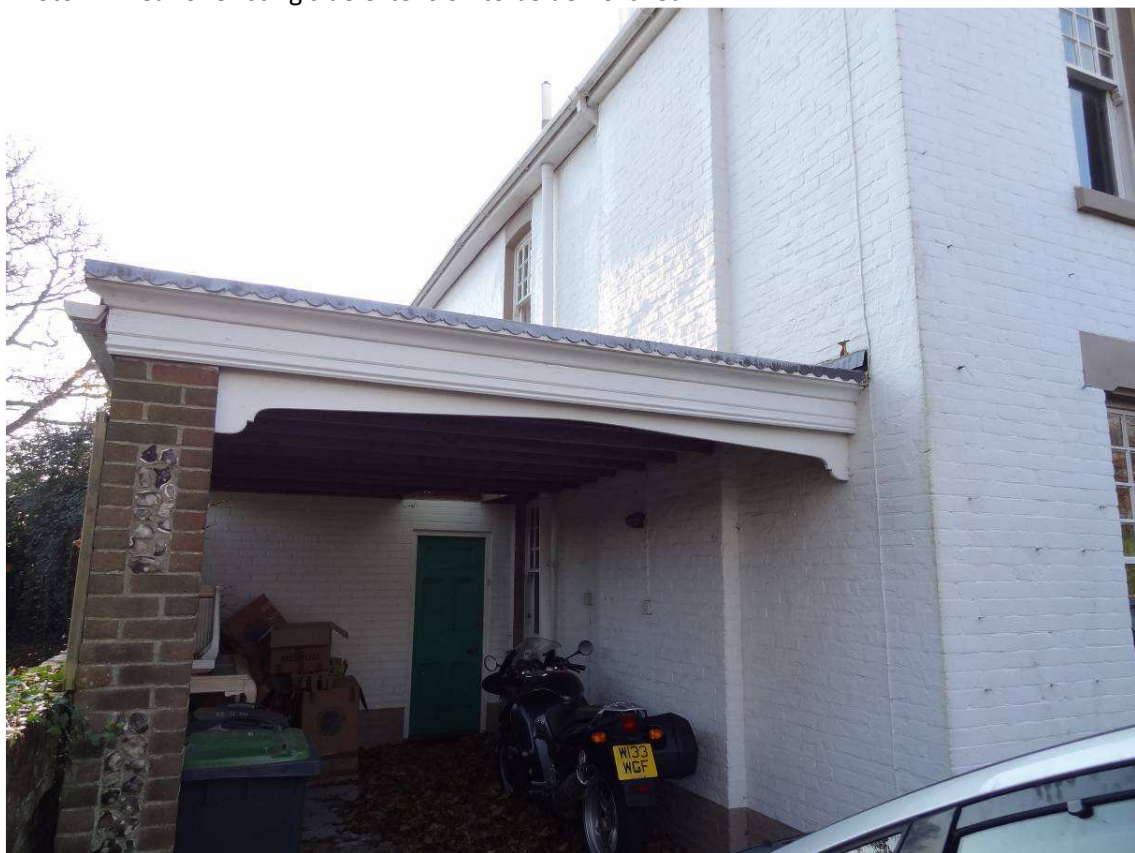
Photo 8 – View of front elevation of side extension from drive.
