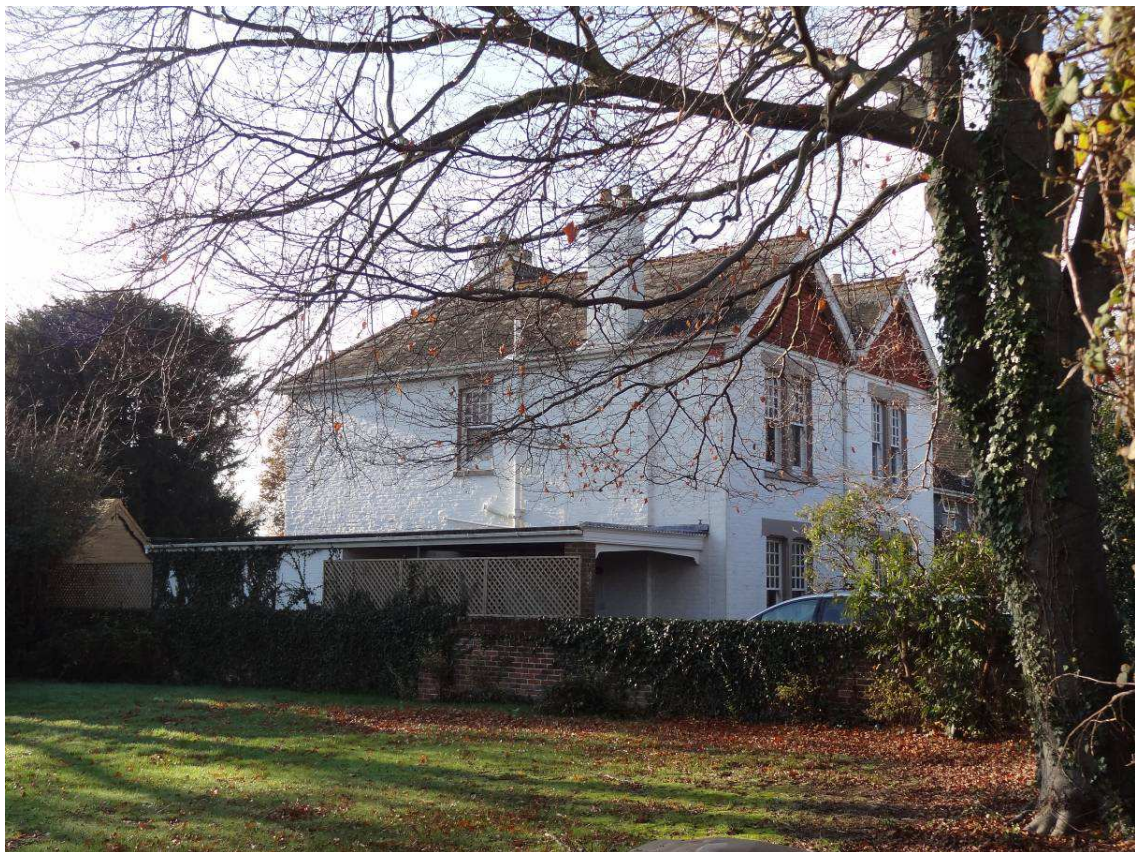
Photo 4 – View from drive entrance of No. 26 showing existing side extension.
