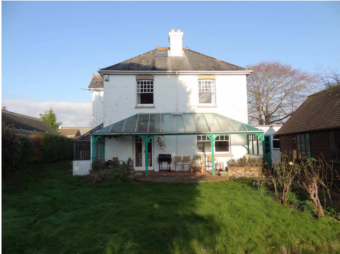
Photo 5 – View of rear elevation from garden. Side extension and outbuilding to right.
