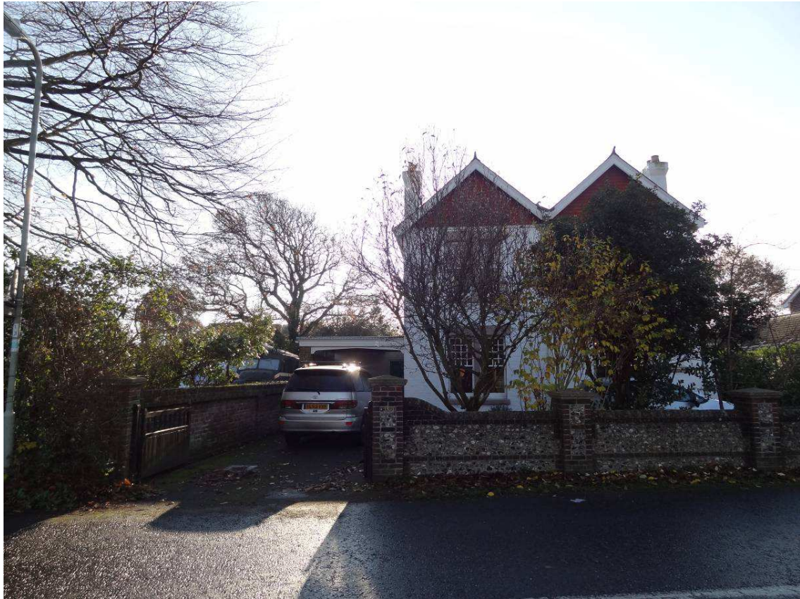
Photo 1 –View looking south across Hollow Lane. Side addition to be demolished left of centre.
