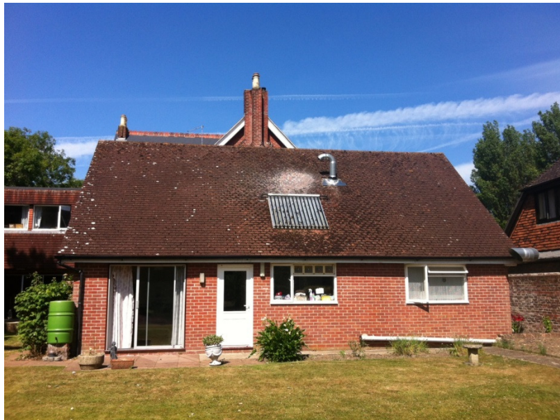
Image 5: Existing kitchen extension, to be demolished
