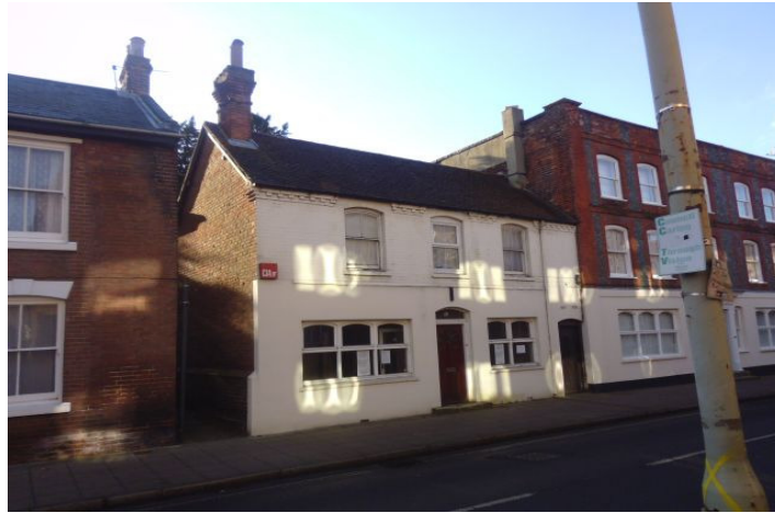
Fig 1: View looking south; East Street
