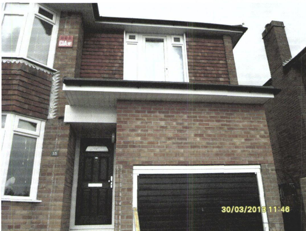
2. Existing Flat Roof Over Garage
