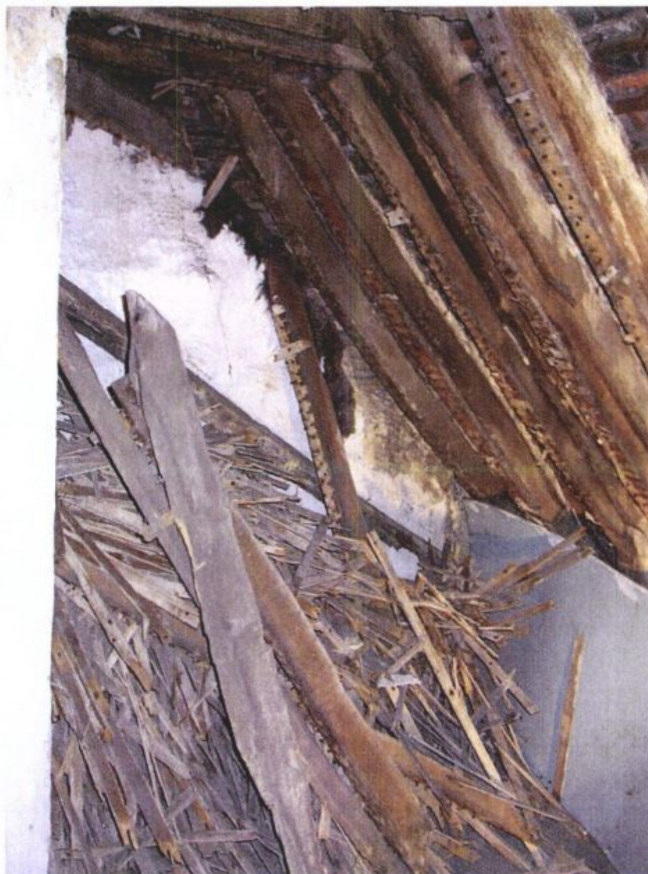
Photo 002 – East Party Wall in Roof Adjacent Stack.
