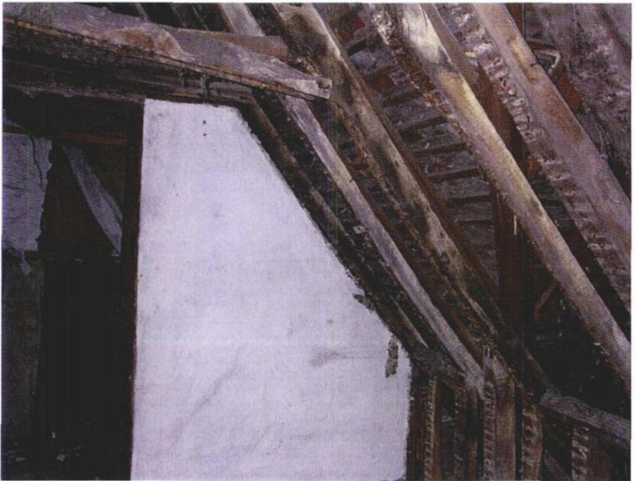
Photo 009 – Roof Accommodation Area. N.W. Corner Showing Stair Wall Panel and Rear Pitch.
