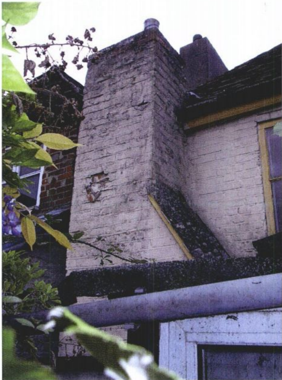
Photo 037 – North Elevation. N.E. Corner Stack.
