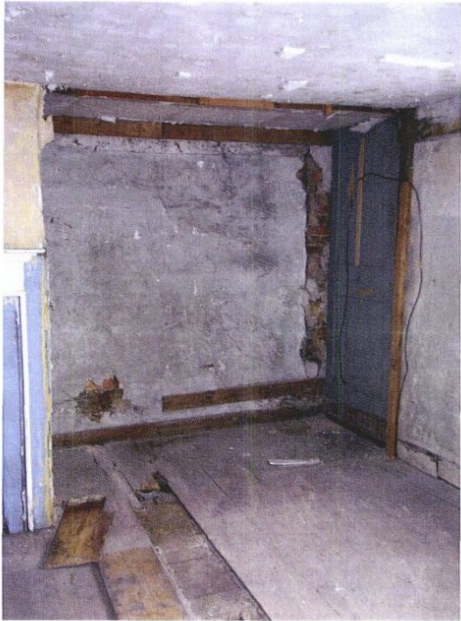
Photo 028 – Bedroom 2. S.E. Corner. Showing East Party Wall.
