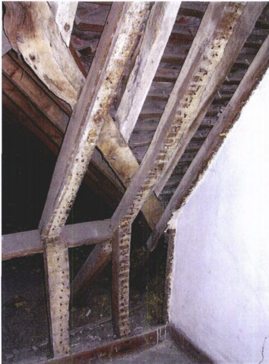
Photo 005 – Roof Accommodation Rear Pitch. Northeast Layboard.
