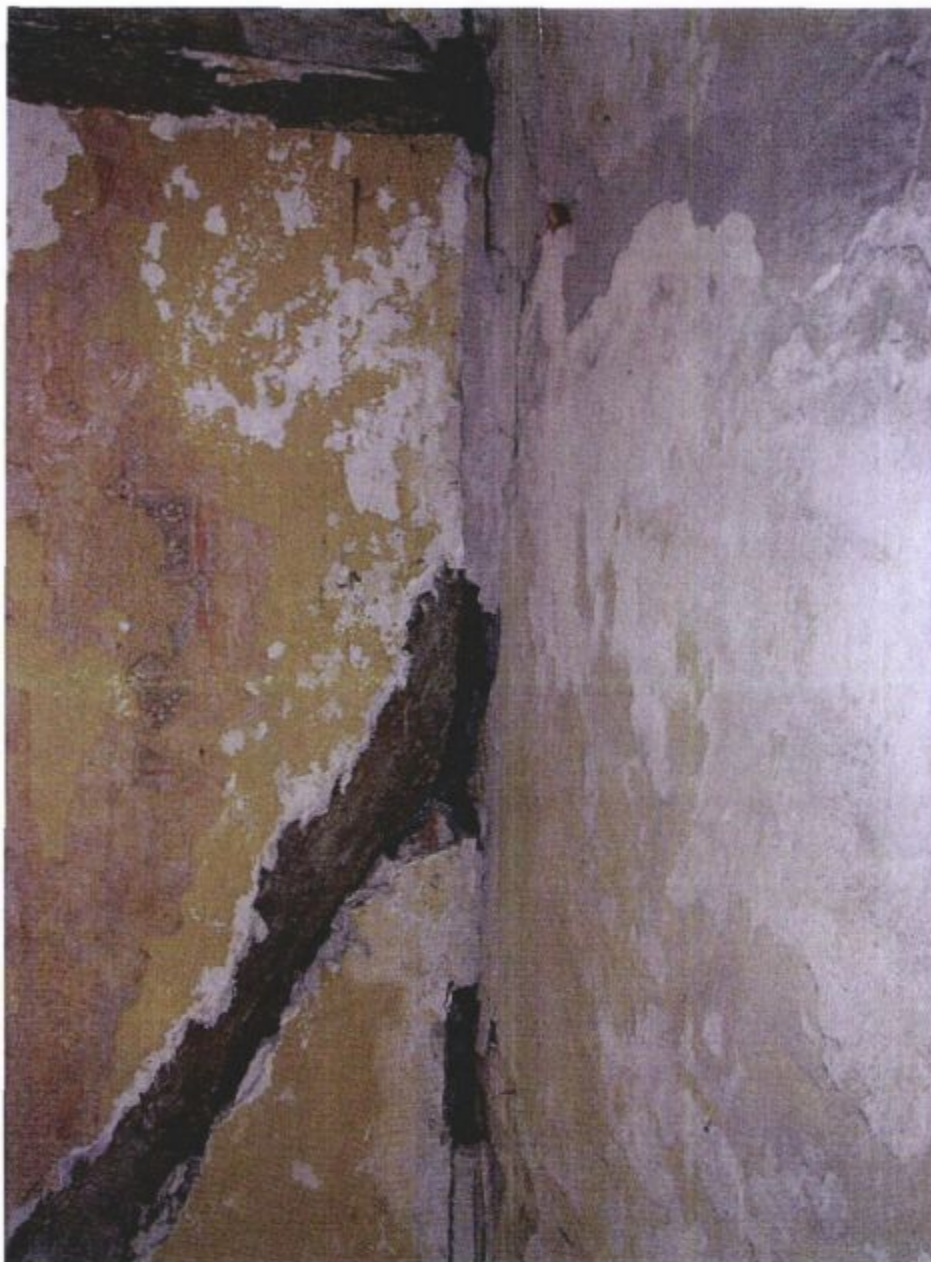
Photo 019 – Bedroom 1. S.E. Corner. Partition/South Wall Junction.
