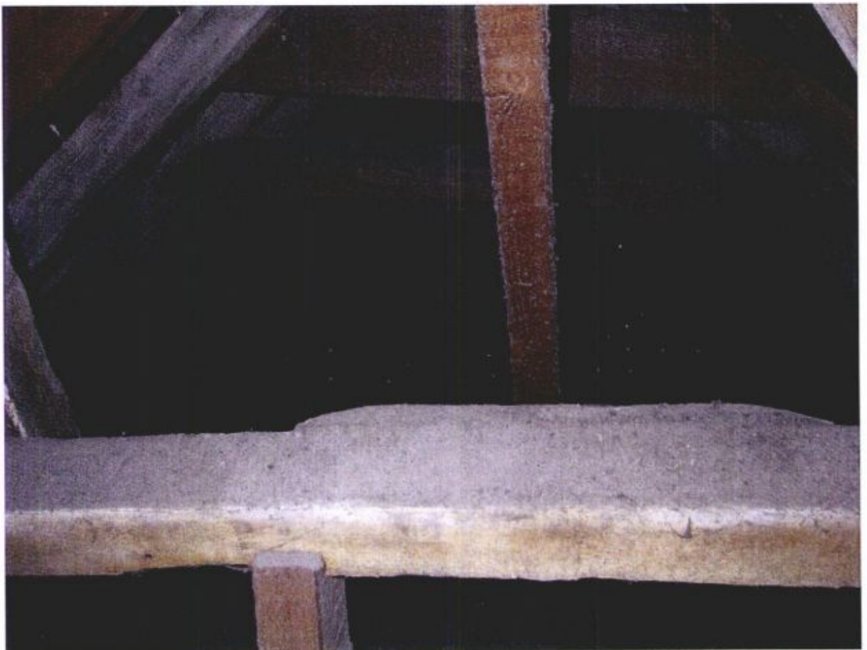
Photo 015 – N.W. Rear Roof Space.
