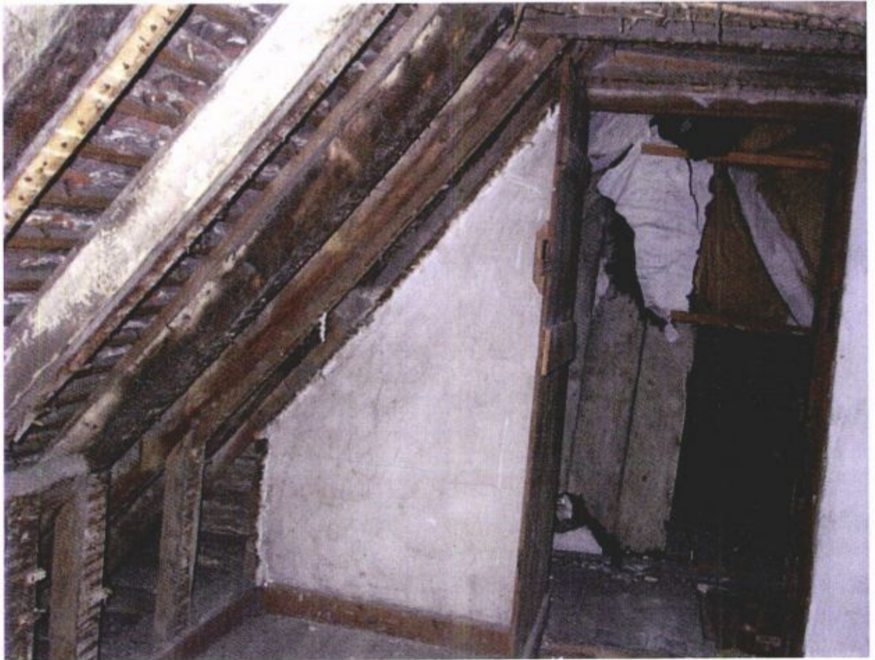
Photo 010 – Roof Accommodation Area. S.W. Corner, Front Pitch.
