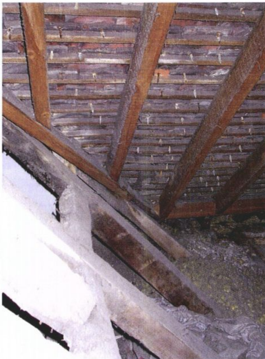
Photo 007 – Rear West Pitch behind Roof Accommodation Area.
