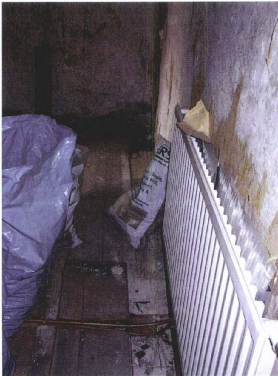
Photo 025 – Corridor. West Party Wall/Bathroom Loadbearing Partition.
