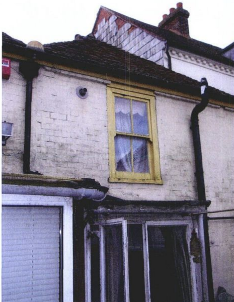
Photo 035 – North Elevation. West Side. N.W. Hip/Party Wall to No. 88.
