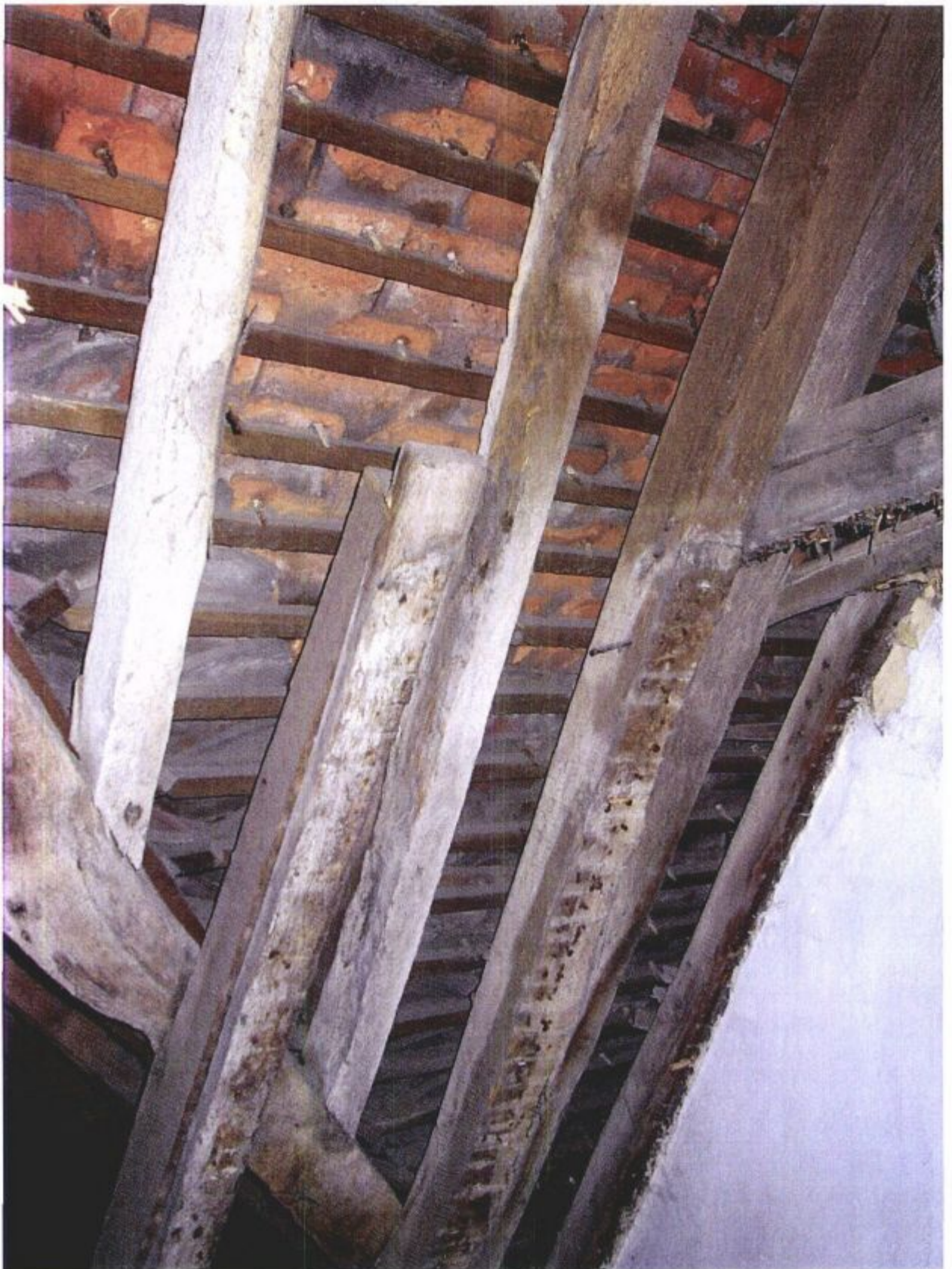
Photo 004 – Roof Accommodation Area. Rear Pitch Northeast Layboard/Beam.
