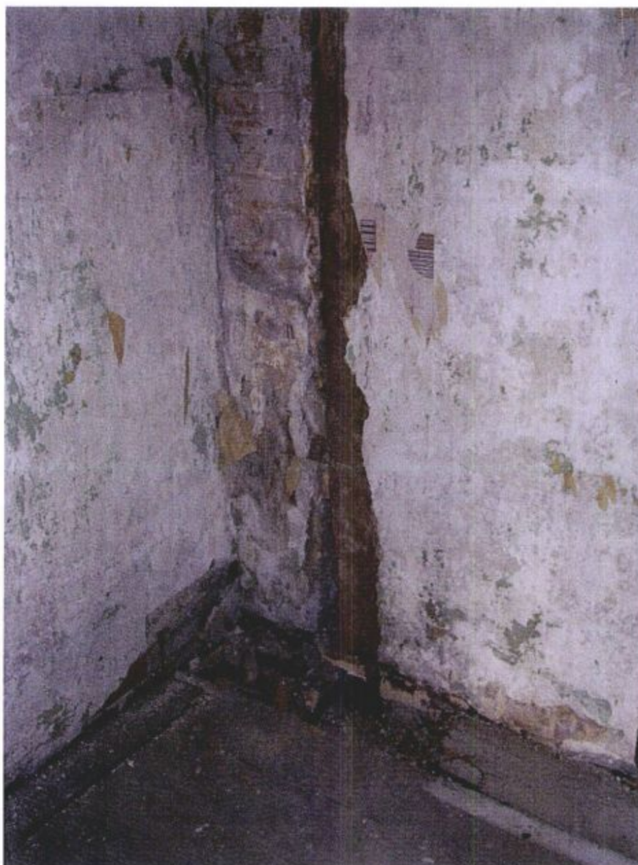
Photo 024 – Corridor. West Party Wall Junction with Loadbearing Timber Framed Bathroom Wall.
