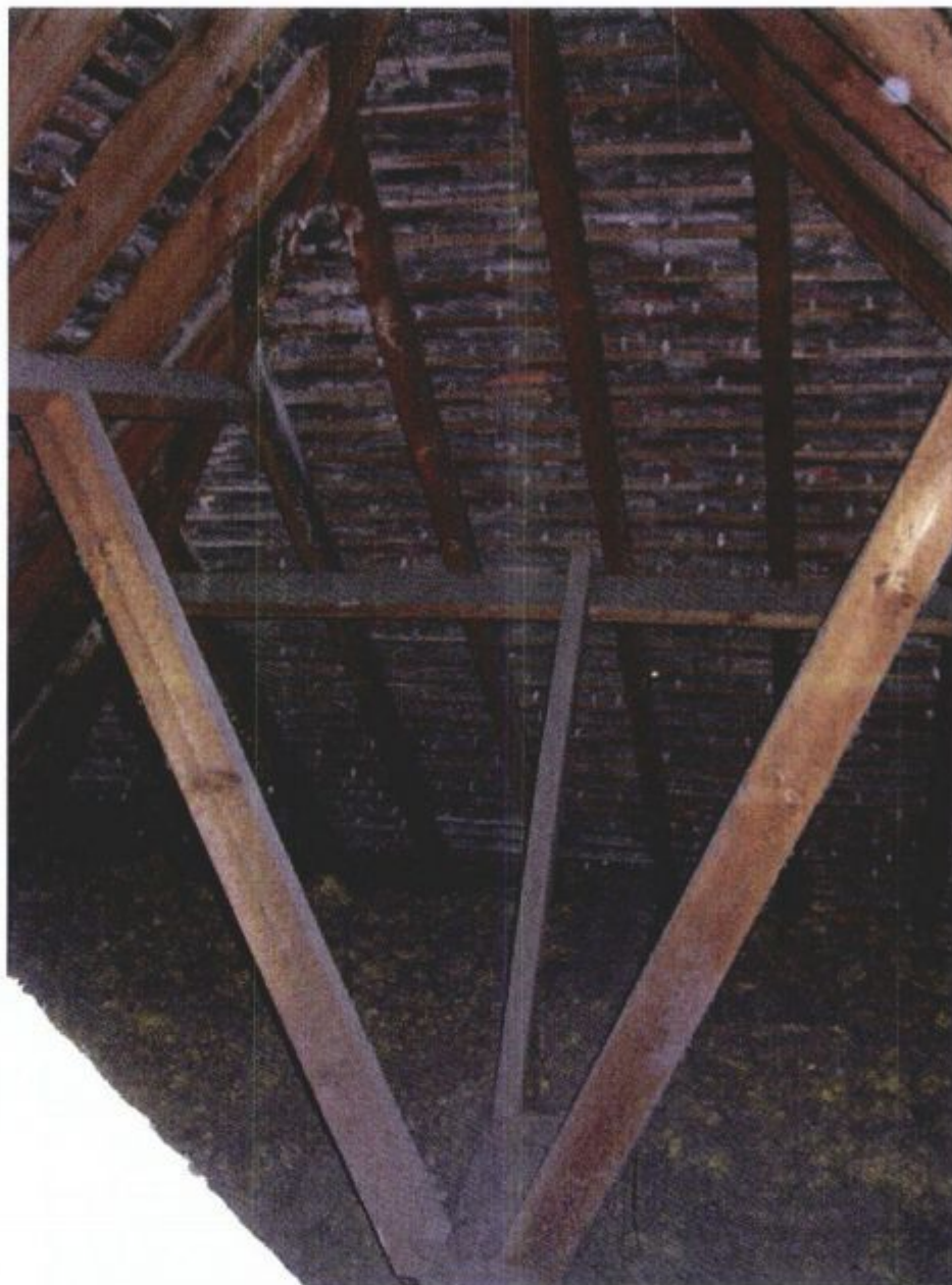
Photo 006 – E-W Roof behind Roof Accommodation Area.
