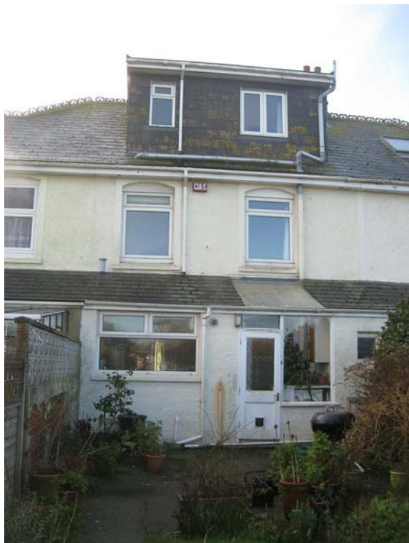
REAR VIEW (NORTH)
