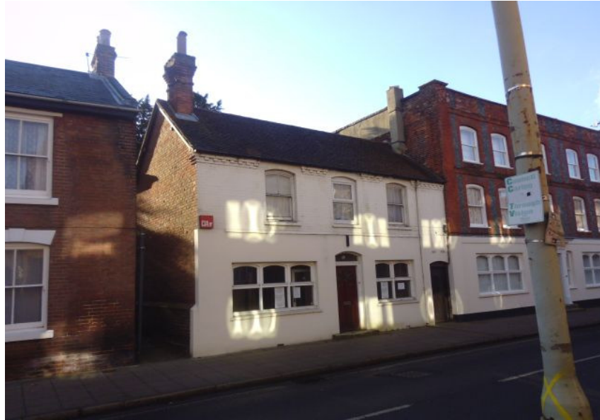
Fig 1: View looking south; East Street
