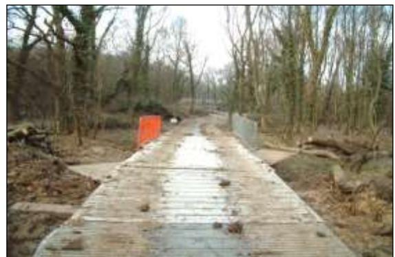
Photo 12: Custom designed sectional tracks can be joined to support very heavy traffic use through sensitive areas.
