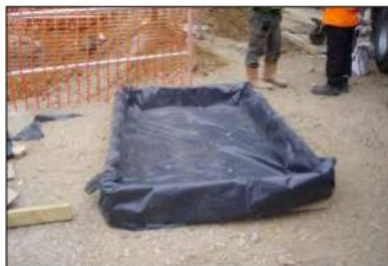
Photo 47: Soil bunding or a supporting framework covered in heavy-duty plastic sheeting is essential where there is a risk of spillages contaminating RPAs.
