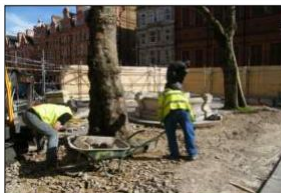
Photo 22: These trees had impermeable surfacing right up to their trunks, which had to be removed by hand before installing new structures.
