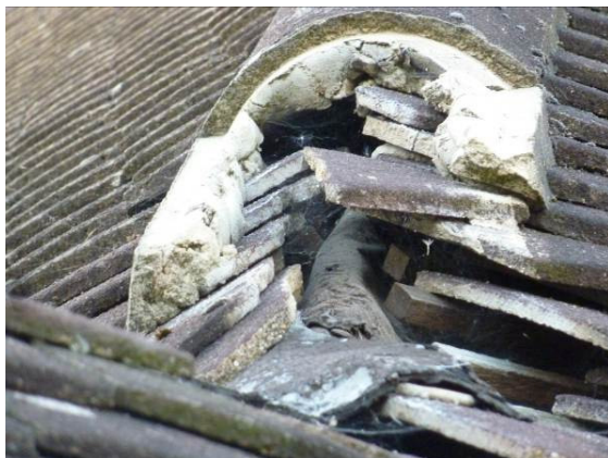
Gaps in roof of rear extension
