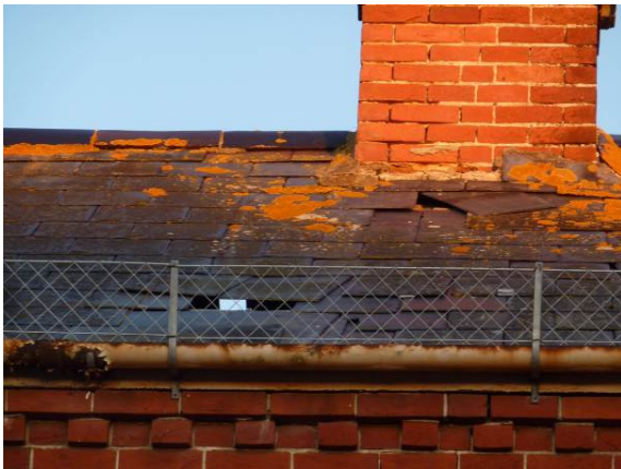
Gaps in roof of rear extension
