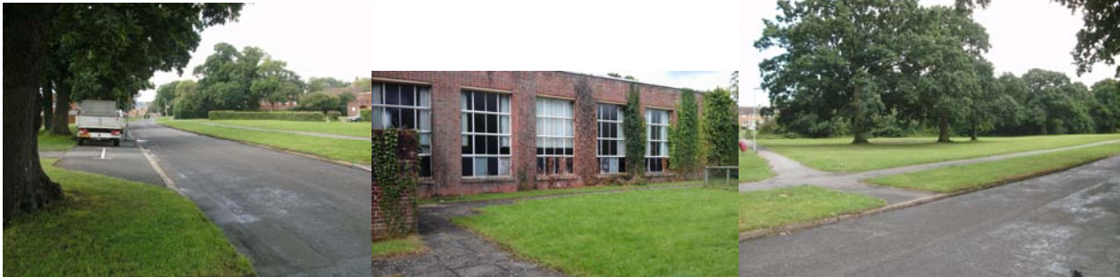
Views of the surrounding site
