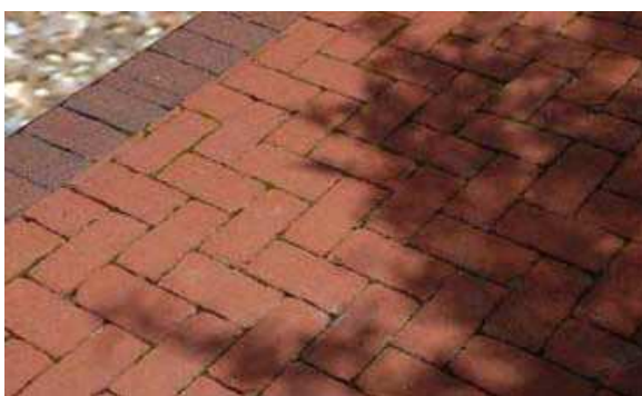
Herringbone pattern block paving with brick edges
