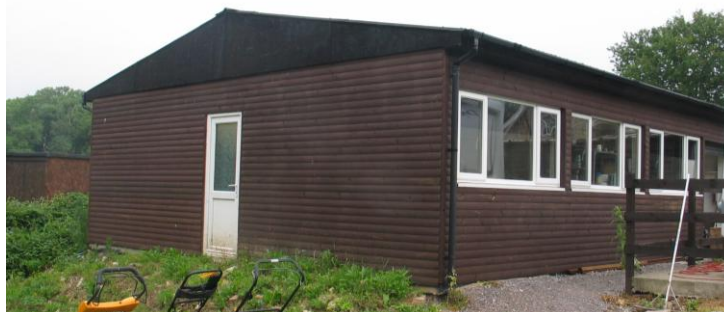
Photo 1 – showing the new building and the materials used in its construction (view from SW)
