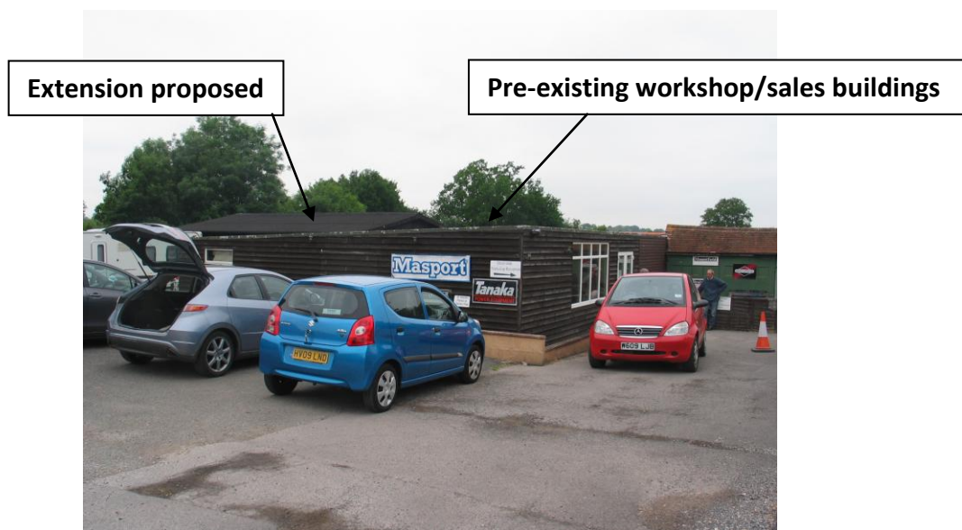
Photo 3 – showing the relationship of the new workshop to the original buildings on the site.
