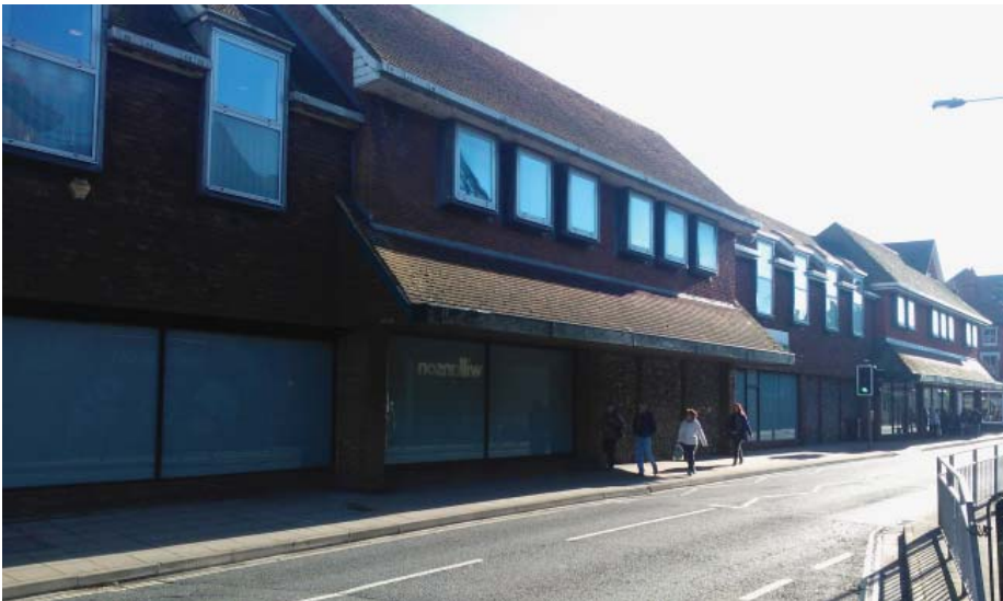
Photograph of Existing Canopies
