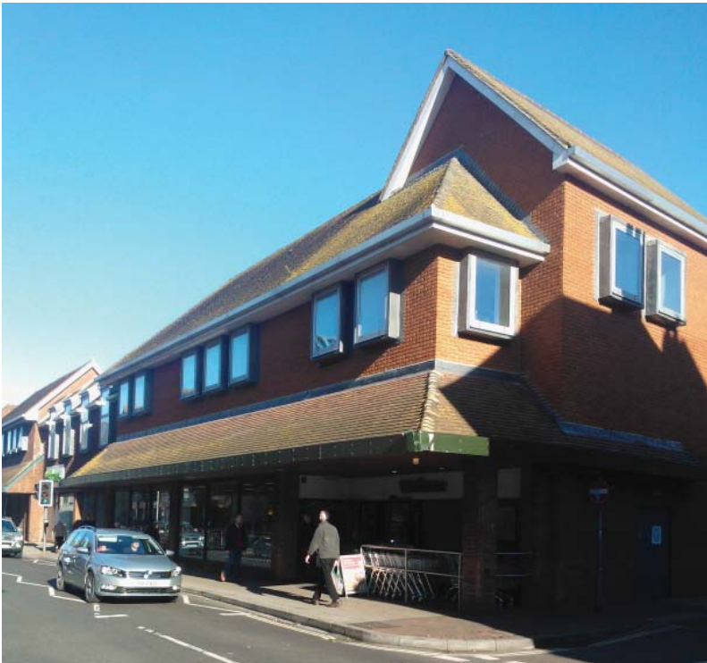
Photograph of Existing Canopies
