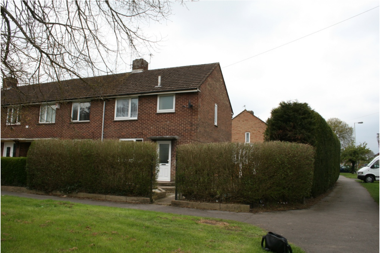
Existing No. 67 Bondfields Crescent
