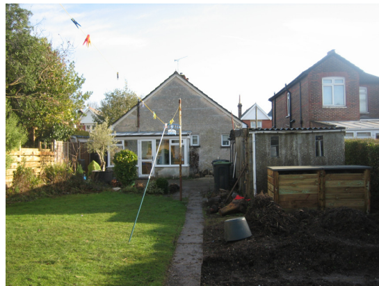
Fig 4. Existing rear elevation, garden and garage structure
