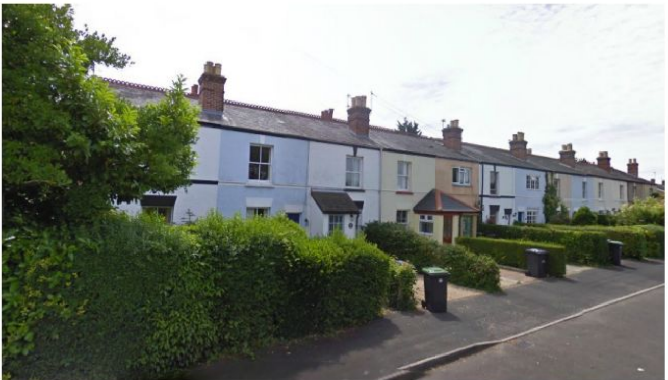
Terrace homes along Kings Road opposite site
