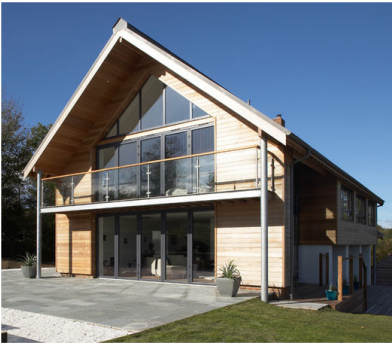
Balconies with overhanging eaves
