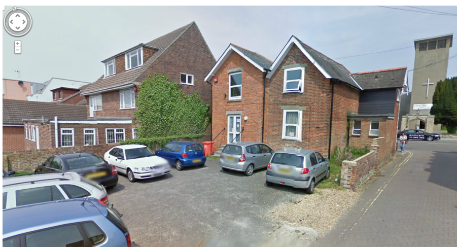
View from the West looking to the rear of site from Portland Road
