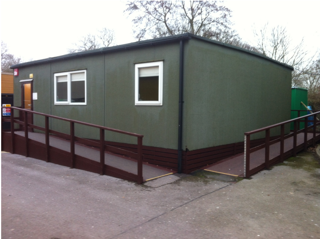
Cabin M – from the south west
