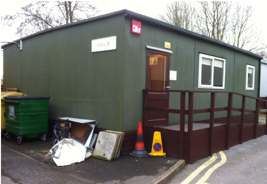
Cabin M – from the north west
