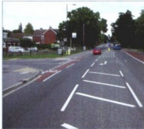
Photo 11 - Protected right turn. The application site is on the left hand edge of the photograph
