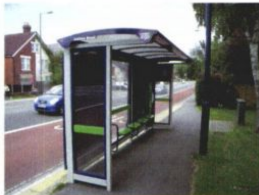
Photo 5 - Southbound bus shelter
