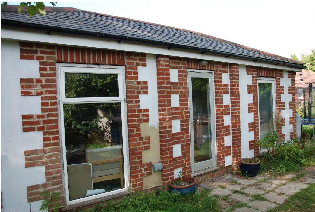
Figure 2 - Brick and render finish to be retained in new bungalow
