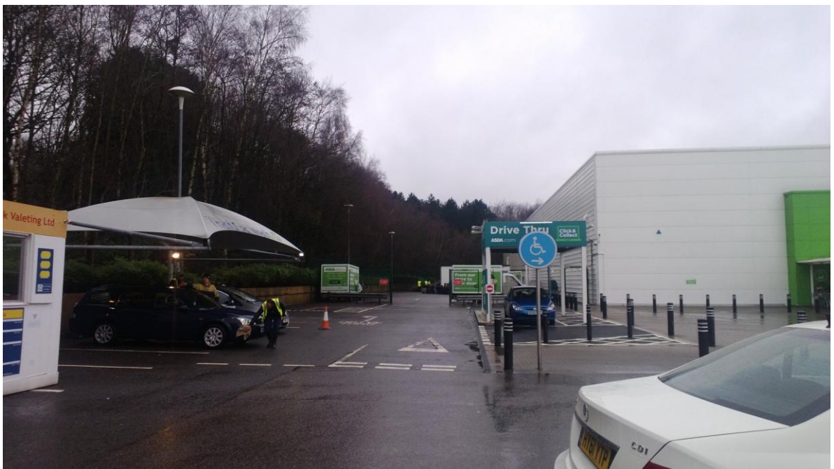
Photo 2. Showing screening of site
