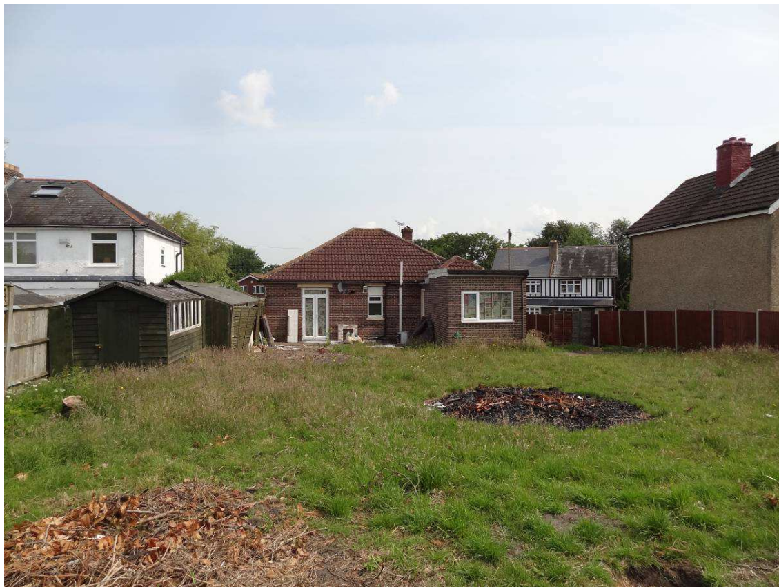
Photo 13 – View from rear garden towards the bungalow with Nos. 16 & 18 to the left, No. 22 to the right.
