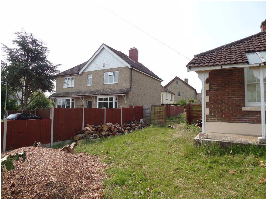
Photo 8 – View of close boarded boundary fence to No.22 (to be retained).
