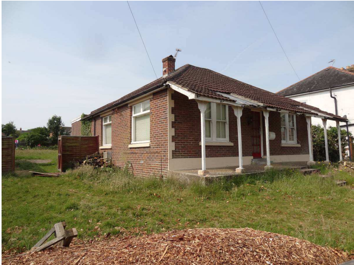
Photo 7 – Close up view of the bungalow at No.20 to be demolished.
