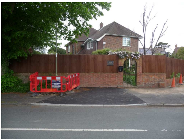
Recently installed drop kerb access on Castle Ave
