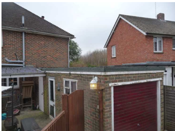
View of Rear extension area (looking South West)
