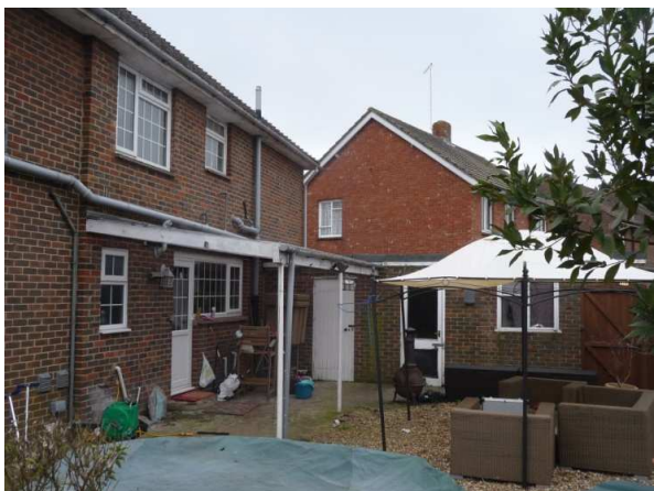
View of Rear extension area (looking West)
