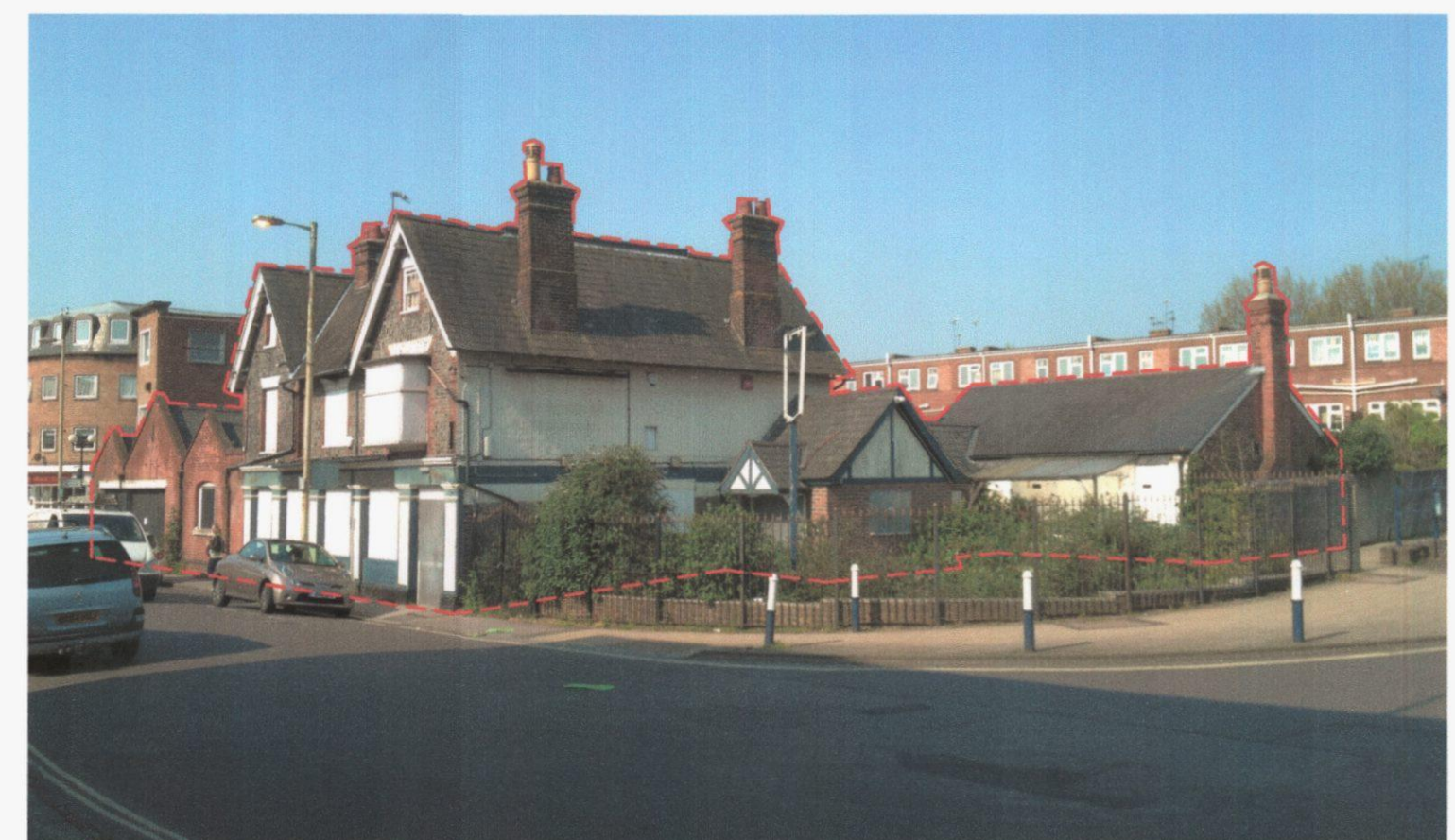
Existing Star Public House viewed from the Railway access road
