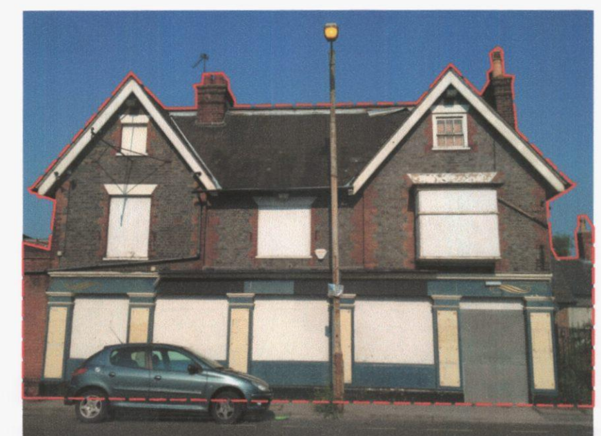
View of the existing Star Public House along North Street
