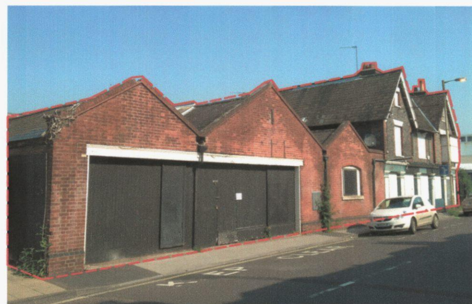
View of the existing Star Public House along North Street
