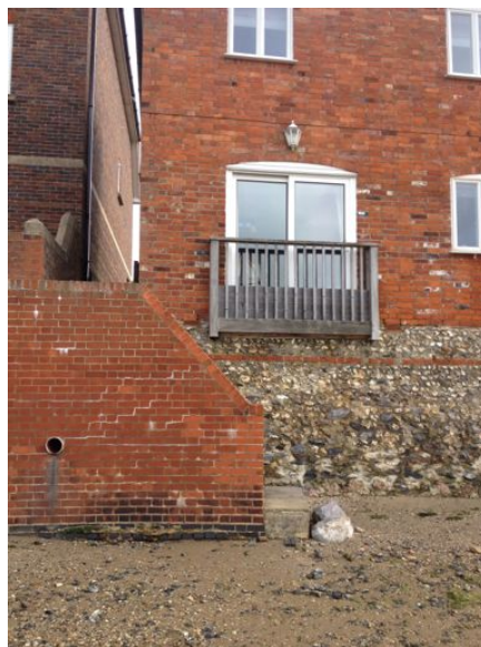
Existing balcony and steps
