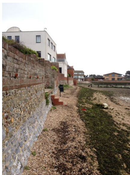
Existing Bin and steps
