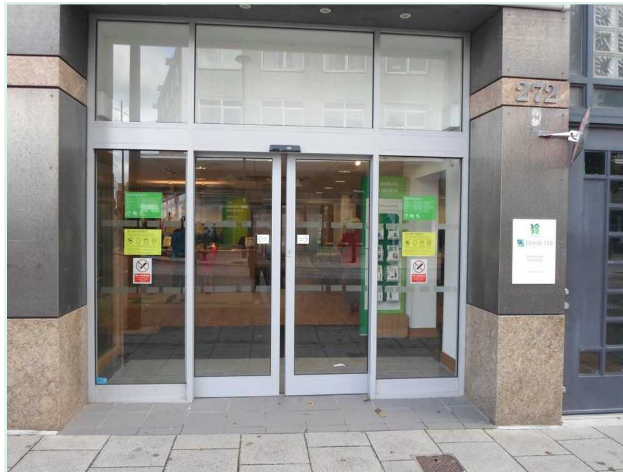
EXISTING SIGNAGE OVERVIEW
