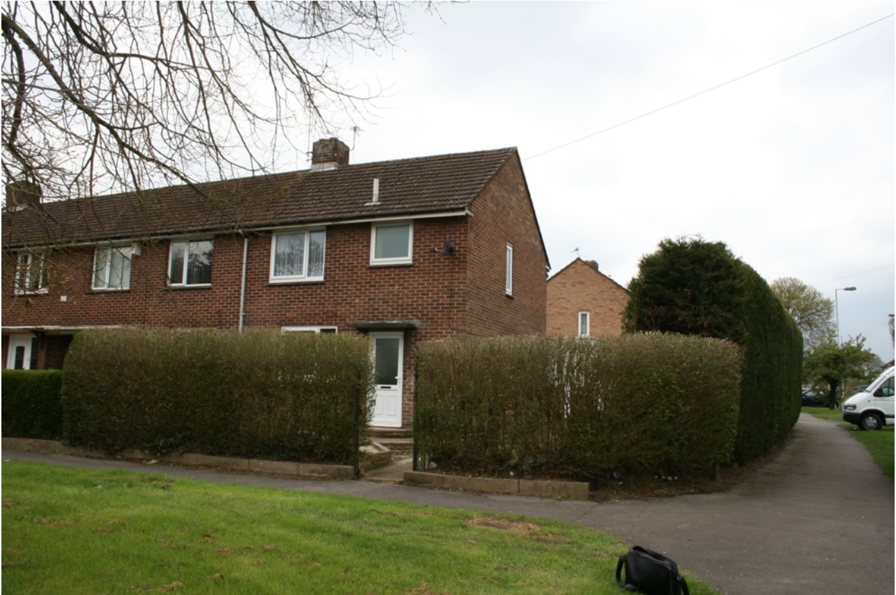
Existing No. 67 Bondfields Crescent
