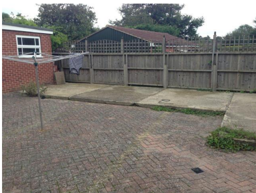
Alternative View of Concrete Hardstanding showing Garage looking East
