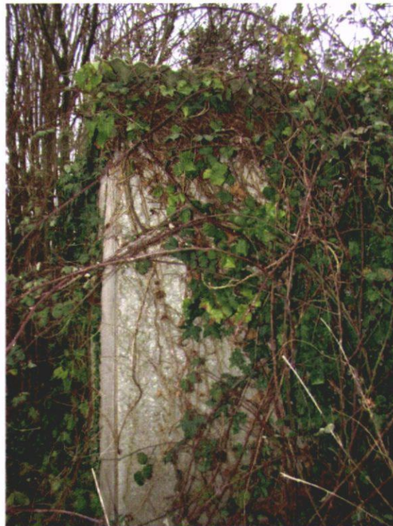
Figure 2: concrete-built single-storey storage outbuilding (B2)
