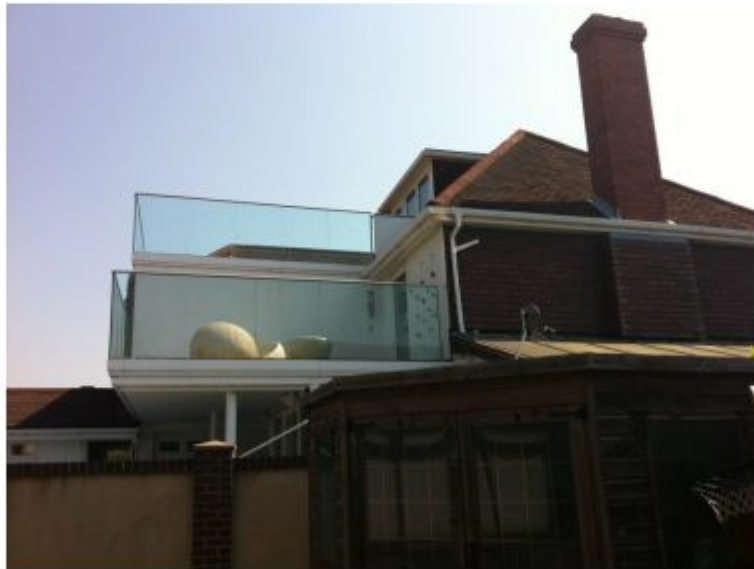
Image 5: Photo showing balconies to rear of No.49
