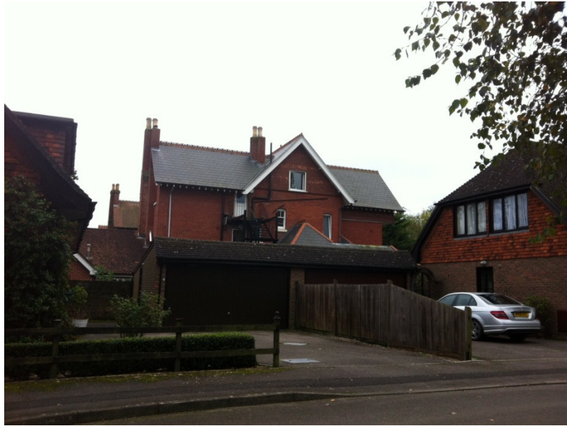
Image 2: View from Silvertrees, showing external fire escape.
