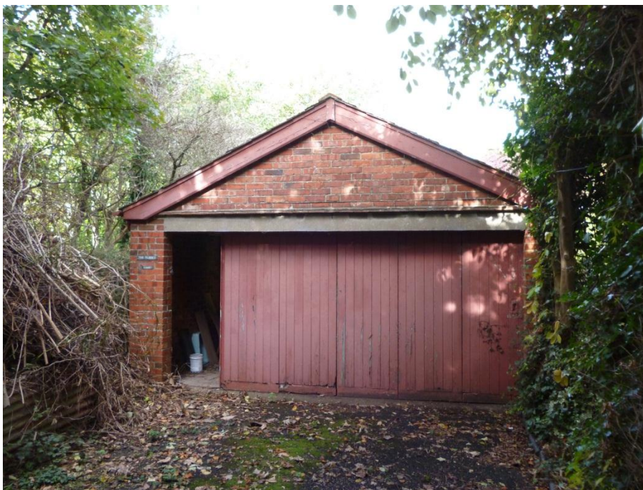
Figure 1: View of existing building from Montgomery Road
