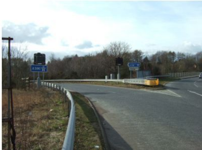
Figure 7. Crash Cushion at A3(M) Junction 3 Southbound On-slip
