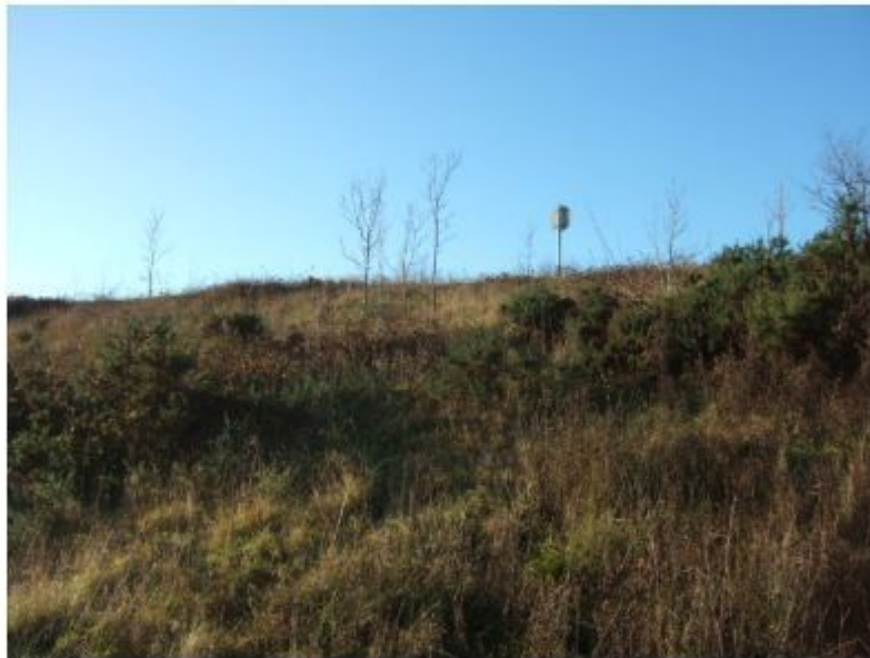
Figure 12. View from the bottom of the Embankment to the A3(M)
