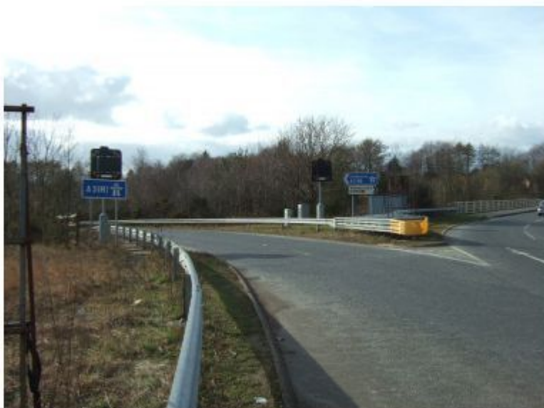
Figure 2. Crash Cushion at A3(M) Junction 3 Southbound On-slip
